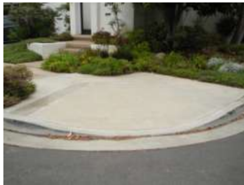
ADA Compliant Curb Ramp meeting current standards
